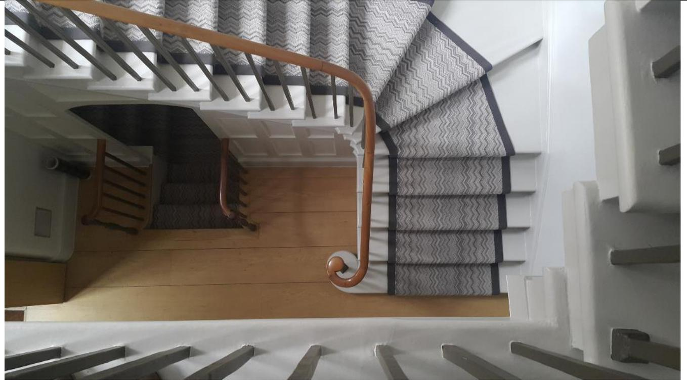
**Photograph 1** – view from first floor landing of the ground floor base of the staircase, showing also the existing (modern) stub stair flight down to the lower ground floor that would be removed.
